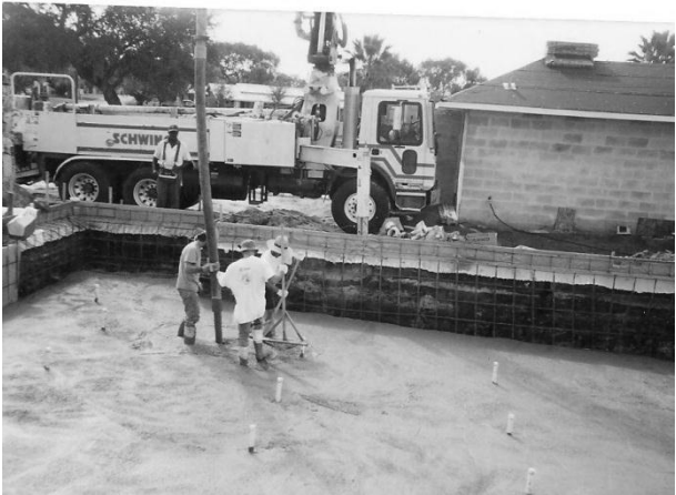
New Pool Construction
