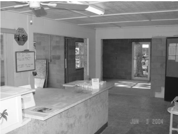
Golf Clubhouse Construction
